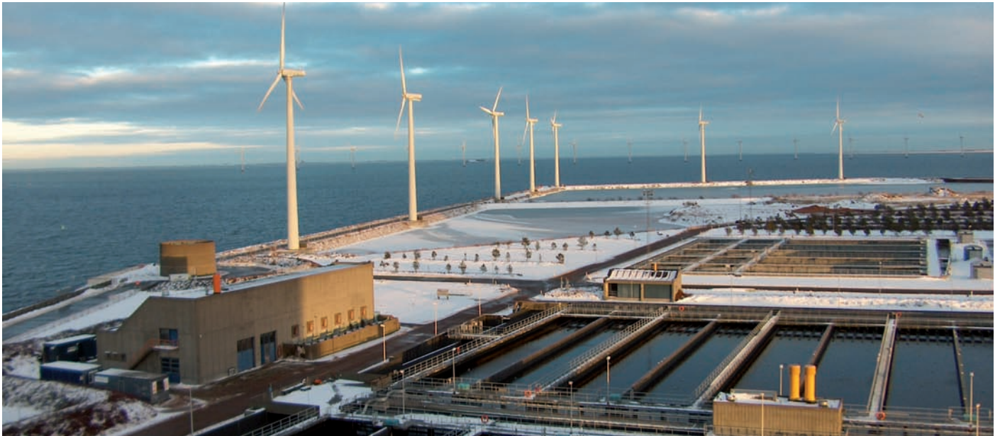
The two plants treat 75-100 million m 3 of waste water from industry and households every year. This is the equivalent to the waste water from waste of 1.1 million people.
